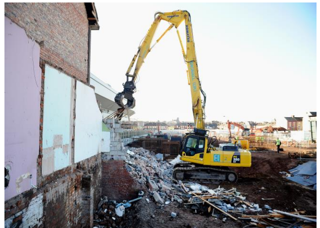
Image: A crane demolishes a building on site
